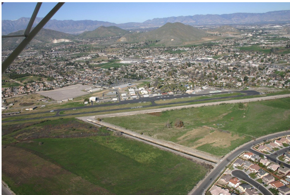
Figure A-10 Flabob Airport, Looking North
